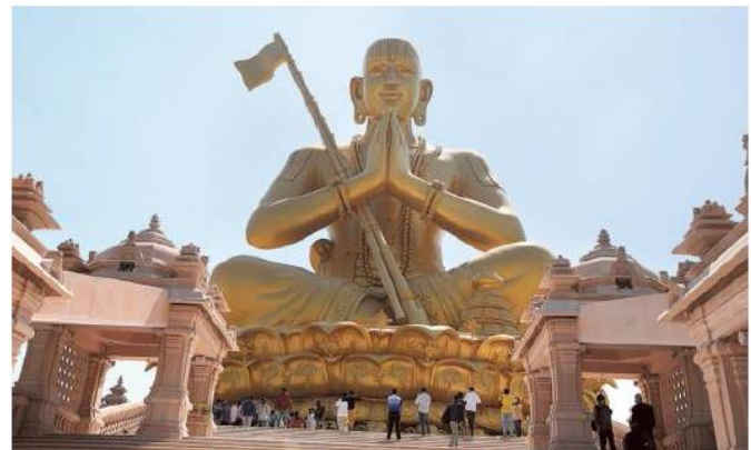
The 1,800-tonne panchaloha statue of Sri Ramanuja was made in China and assembled onsite. THE HINDU
