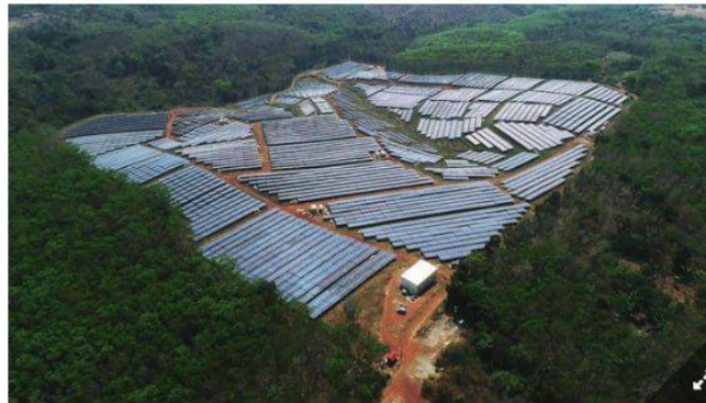
A panoramic view of CIAL's solar plant at Payyanur
