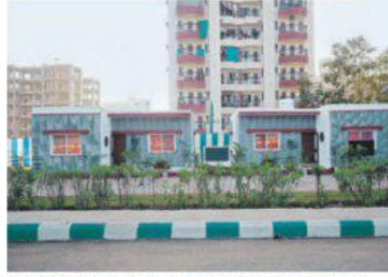
The use of 3D printers by the Indian military is, however, not confined to houses alone.
