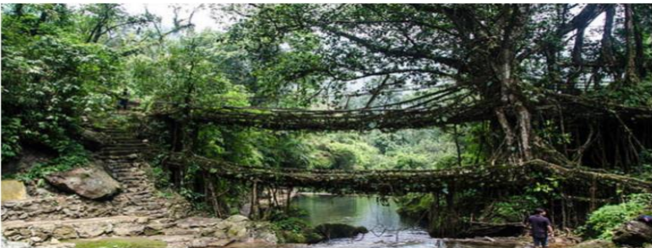
These bridges facilitate connectivity and disaster resilience in more than 75 remote villages in and near the wettest region on the planet. (Source: Wikimedia Commons)
