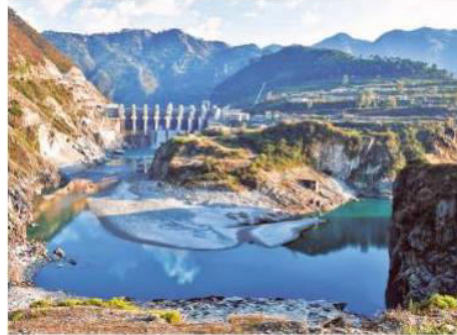
New norms: Environment clearance is mandatory for projects beyond a certain size. • FILE PHOTO
