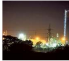
The RFCL plant, during trial production, in Telangana's Ramagundam.
