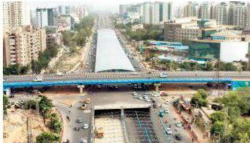
The 22-km-long corridor from Gurugram to Sohna was opened to the traffic on Monday •SPECIAL ARRANGEMENT
